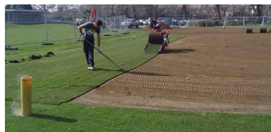
Where time is limited, grass can be established by turfing although this is more expensive
