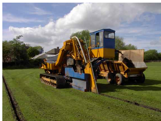
Installing pipe drainage in a new pitch
