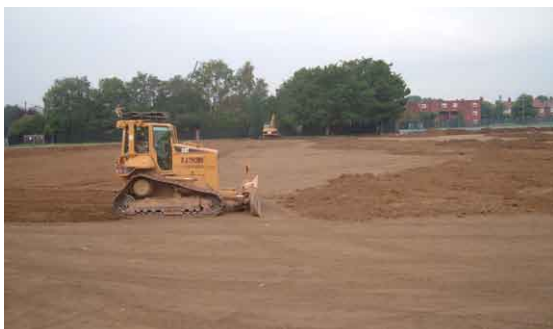
To create a level surface, it may be necessary to strip the topsoil, regrade the subsoil, and replace the top soil
