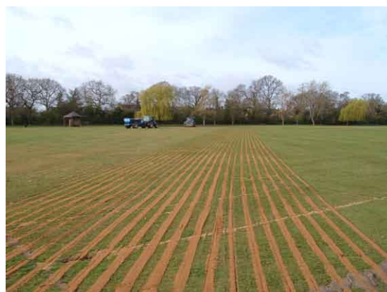
Sand grooves installed at 260 mm centres
