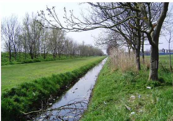
Adjacent water course can provide a convenient means of achieving efficient drainage provided that a 'land drainage consent' can be obtained
