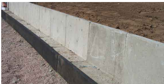
Pre-formed ditch channel simplifies construction
