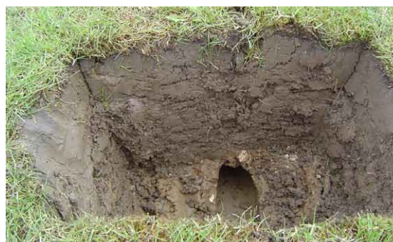
Cross-section through pitch showing a mole channel and leg slot
